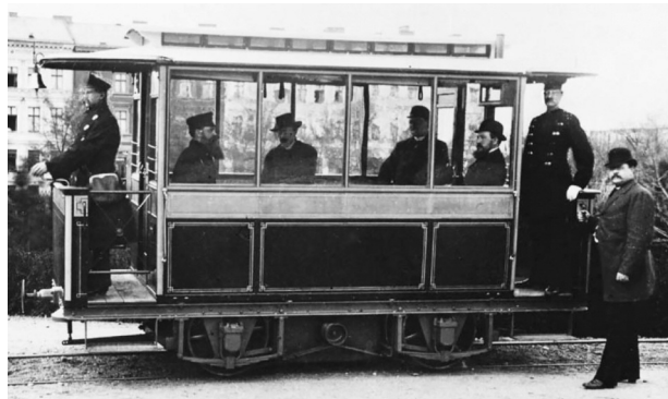
The world's first electric tram began operation in 1881 in Germany and was produced by Werner von Siemens.
